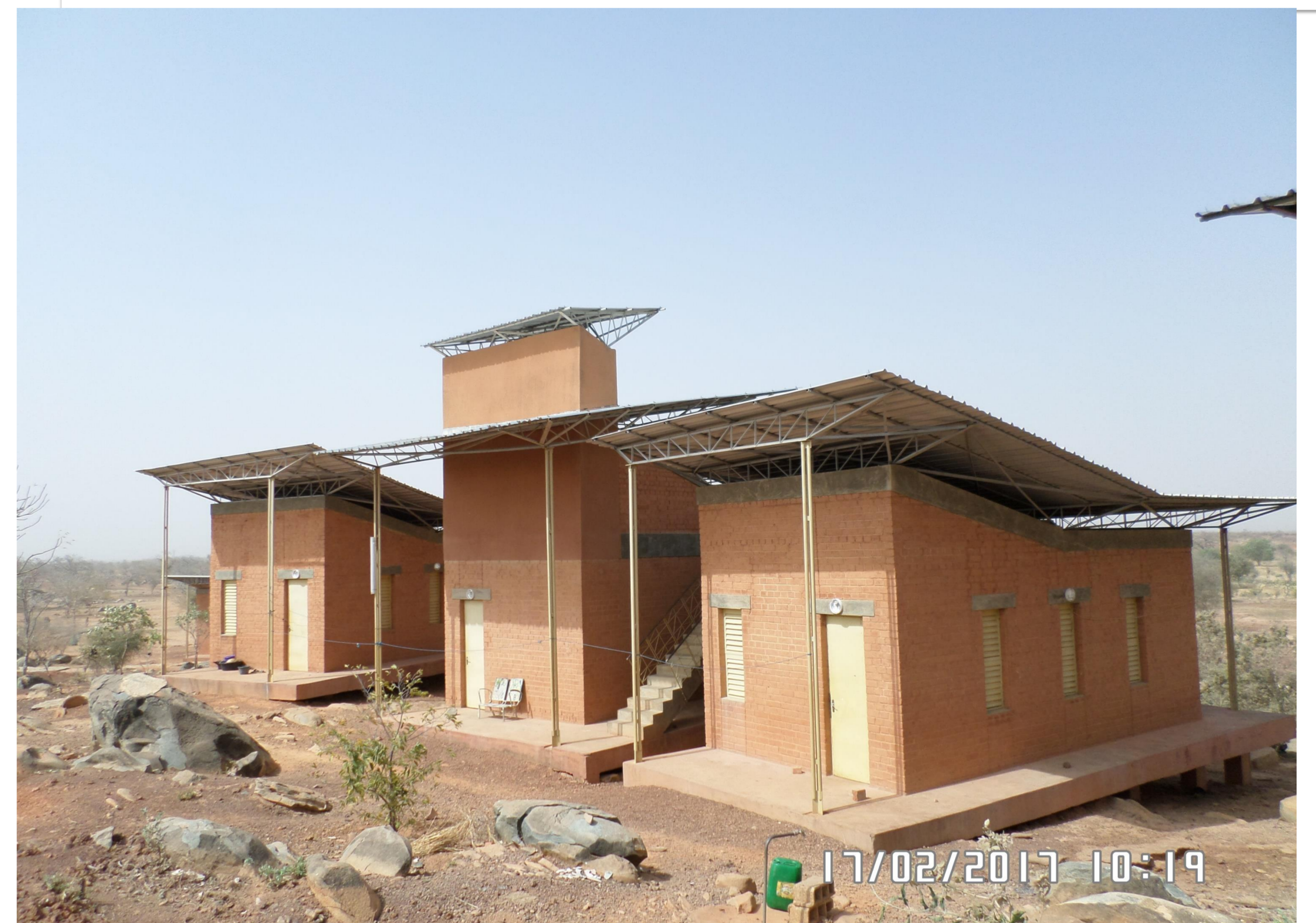
► Fig. 2: Village Opéra de Loango , Architect: Francis D, KERE
